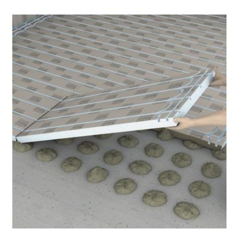
Irregularities in the substrate can be levelled out using the dot technique (possible only for the thickness 50 mm):
